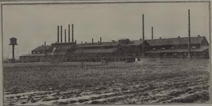
HURON STEEL PLANT
